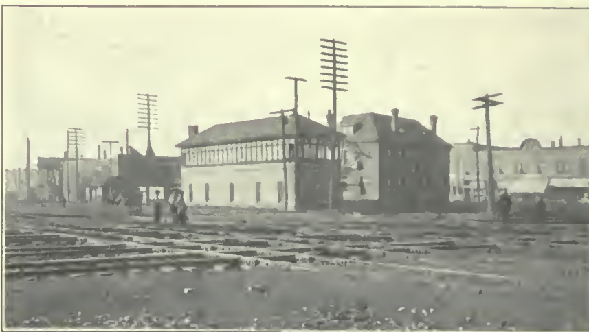
FIG. 260. GRADE CROSSINGS. Burnside crossing of the Illinois Central Railroad with the Belt Railway of Chicago and the Chicago, Rock Island & Pacific Railway.
